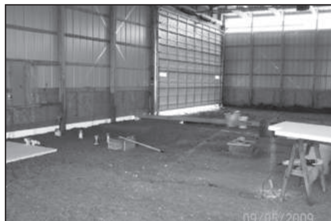
Beginning interior work on the shop...initial plumbing.
