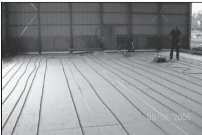
Scott installing tubing for in-floor heat.
