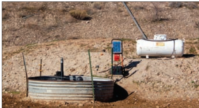
► Left: The gravel pit is electric-fenced with a solar-powered fence charger, while well water is pumped to a pond and is then fed into this stock tank through an underground pipe. The water tank heater is powered by propane.
