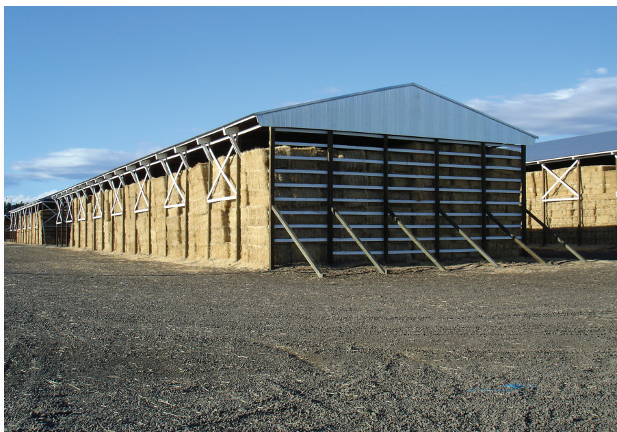
▶ Recommended for storage of new large square bales in high-humidity regions are roofed structures with open sides.
