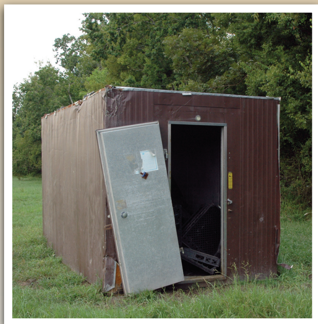
► Above: Louis Pomes has most of the Hurricane Katrina debris cleaned up from his pastures, with the exception of this walk-in freezer and the trash he can't reach in the trees.
