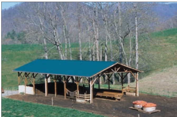
► Winter feed structures combine hay racks, water tanks, concrete pads and manure storage areas.
