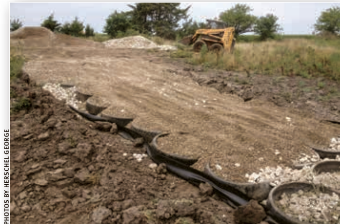
PHOTOS BY HERSHEL GEORGE ► Above: Construction of a pond access ramp using geotextile fabric and tires near Garnett, Kan.
