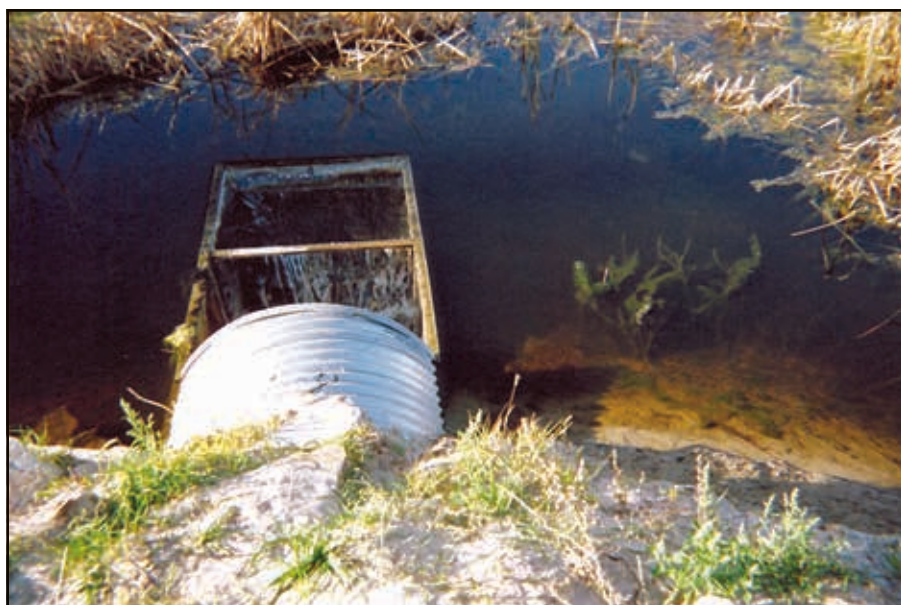
► At the site of a vehicle crossing, a weir was installed on one of the Cedar River’s tributary creeks. Designed to enhance water flow and stabilize creek banks, as well as the crossing, weir construction is an example of Pelster Ranch conservation projects completed in cooperation with the Natural Resources Conservation Service and other agencies.
