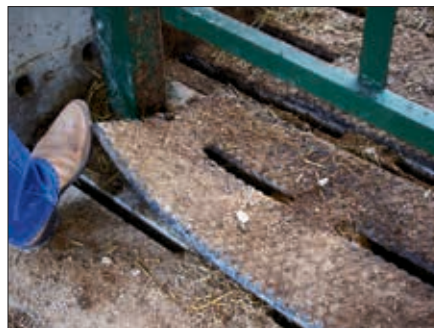
► All of the concrete slatted floors and the area directly in front of the concrete feedbunks are covered with black rubber slats.
