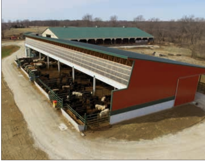
► Above: The higher end of the monoslope faces south, allowing the sun to shine all the way through the barn during the winter.
