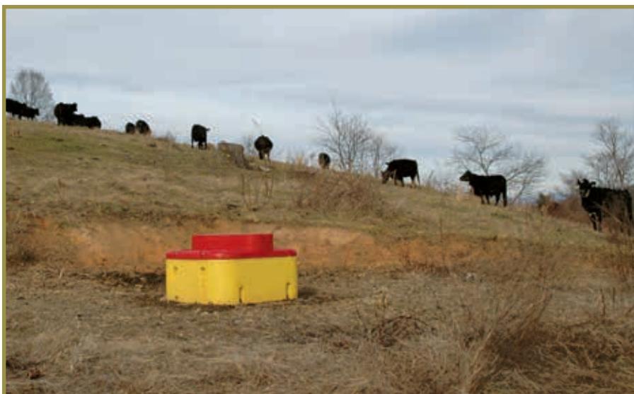
► Below: Bass Hyatt installed watering systems around his farm to keep his cattle out of the creeks.
