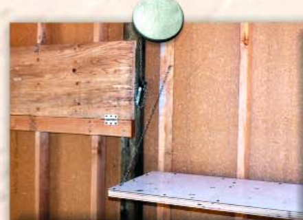
► A board held by hinges and chains (right) serves as a simple shelf for writing or holding vaccination supplies. It can also easily be tucked up against the wall out of the way (left).
