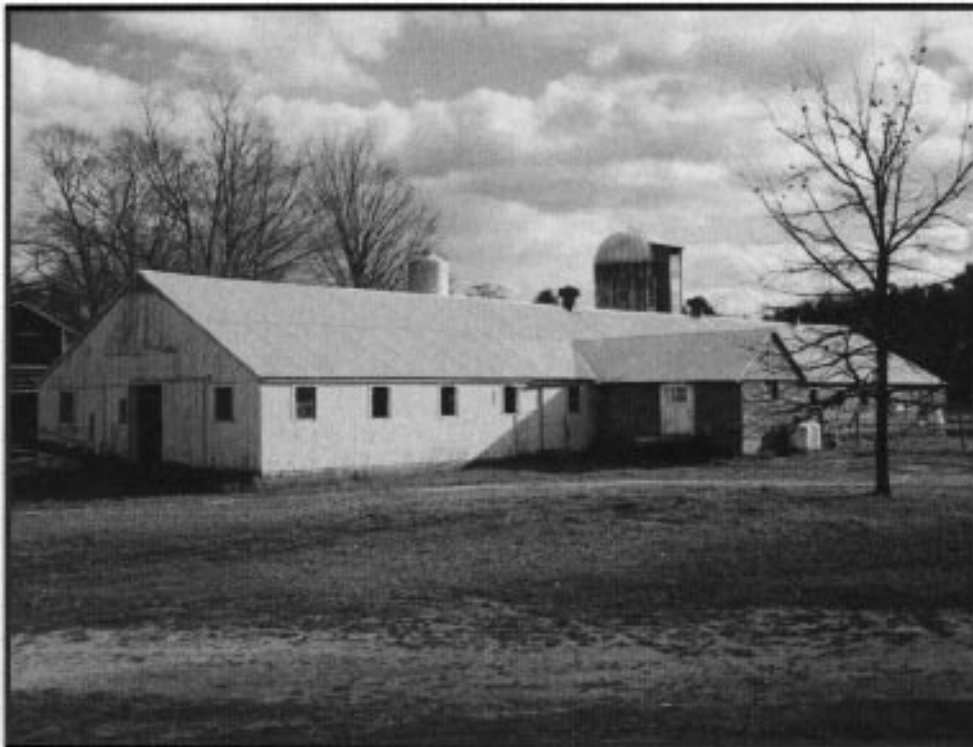
This dairy stanchion barn at Dry Hollow Farm in Massachusetts was recently renovated into a free-tall beef barn. Recycled material, along with improved watering system and handling facilities make this barn more functional.
