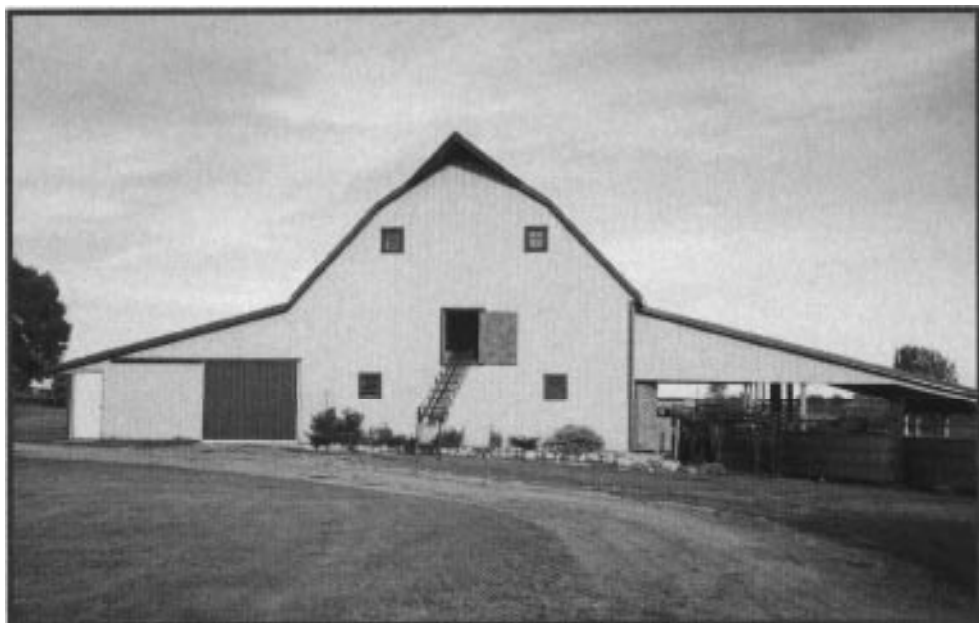
Renovation work on Bar J Ranch's multi-purpose barn was completed in 1995. This 78 x 104 foot facility features calving stalls, a sale ring and cattle handling facilities.
