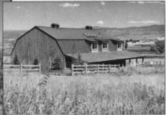
The barn's east side reveals its corrals, dormer windows and skylights. The large, diamond window hadn't been installed on the south wall at this stage.
