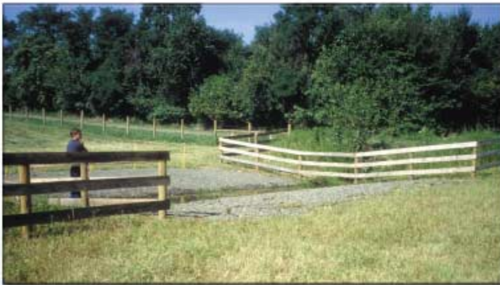
► A newly installed creek crossing prevents erosion.
