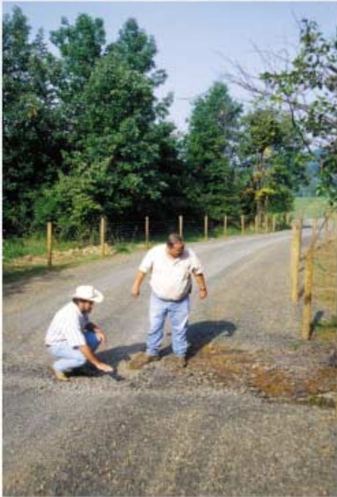
► Although the August heat dried up the stream, hardened crossings limit the cattle's access to the creek and prevents them from damaging fragile creek banks. Wylie is shown with Extension agent Gary Hornbaker.
