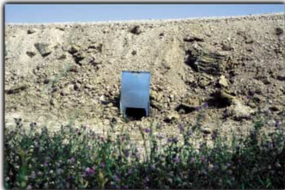
► Protecting water quality requires more than just paying attention to water flow on your own land. Headgates have been installed at drainage points above the Edwards bull-development center to control the flow of water traveling from neighboring fields.
