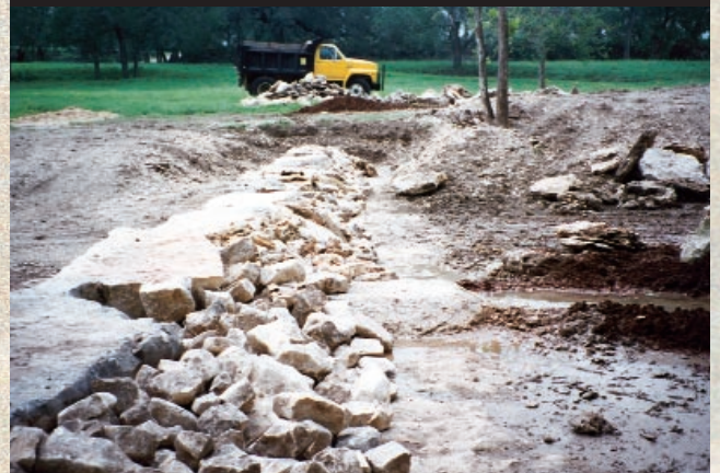
During the severe drought of 1996, Mike cleared gravel out of the creek and built two low-water dams. Then he contoured the slopes above the creek and sprigged them with coastal Bermuda grass.
