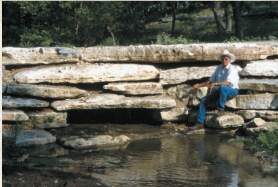
At all creek crossings the Cornetts tried to rock in the banks to prevent erosion. They seeded the disturbed areas with native grasses.
