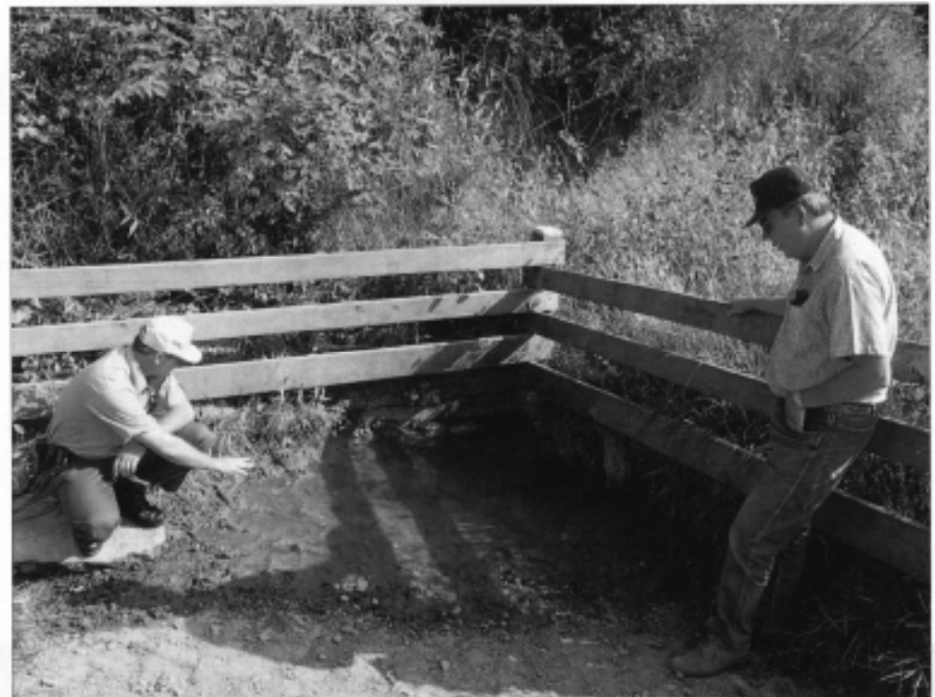
In areas without springs for stock water tanks, water ramps were constructed to allow limited access to water.
