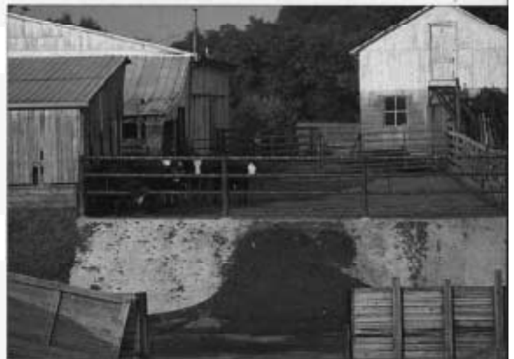
Waste storage areas have been constructed at two of Pletcher's farm feedlots. The structures are designed to hold waste from 200 head for up to 90 days.
