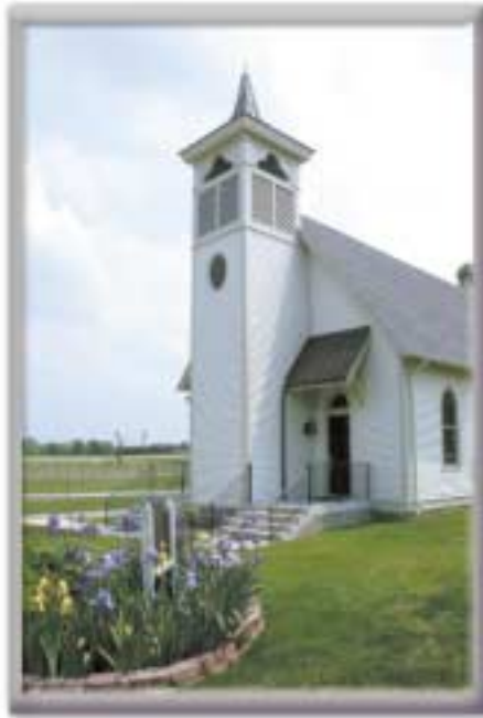
Even though they are not members of Thompsons Station United Methodist Church, the Herons helped fund renovations of the 123-year-old building.
