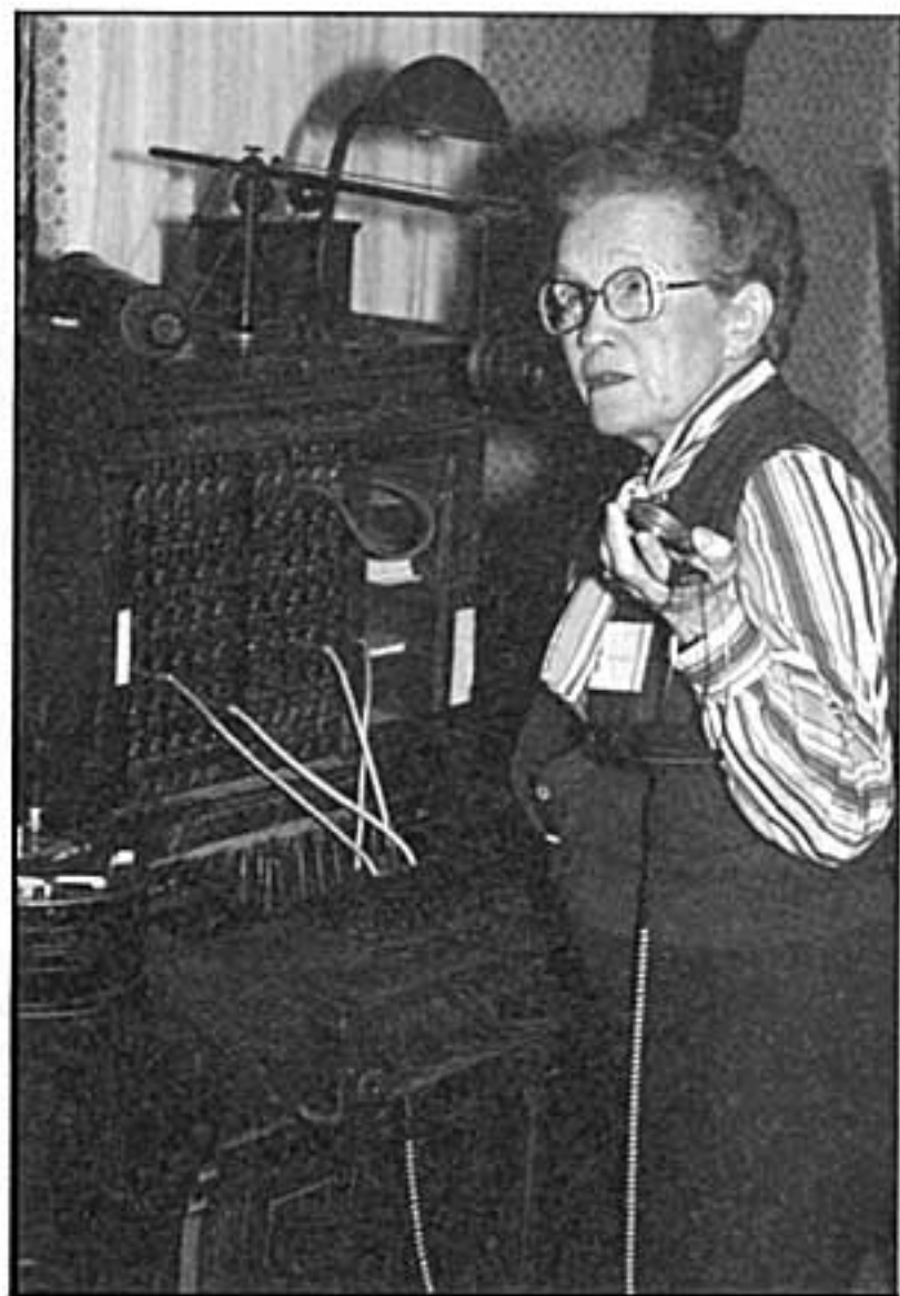
A bucket of sand was kept beside the early switchboards as lightning arrestors were not well-developed and the wires were known to catch fire.
