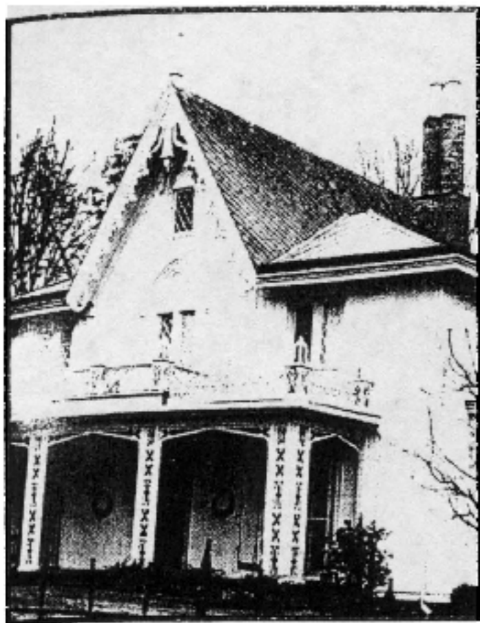
Colonial, Federal, and an architectural style distinctive to the area known as Hudson River Bracketed dot the villages and countryside. The Delamater House in Rhinebeck is labelled American Gothic. Gingerbread and Victorian, even Louis XIV influences can be found in the eclectic mix sprinkled throughout the two counties.
