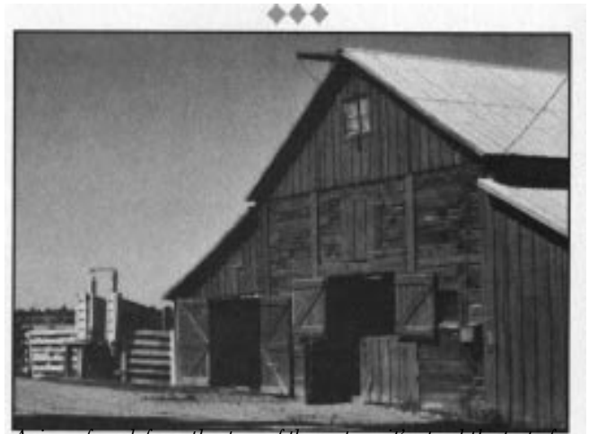
A piece of work from the turn-of-the-century, it's stood the test of time and northern Nevada winters.
