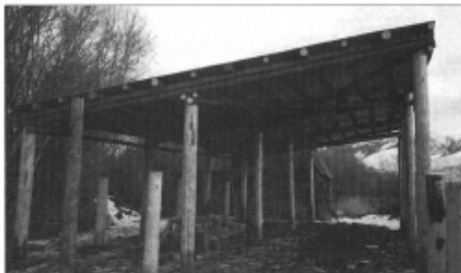
This pole shed provides very inexpensive, but durable protection. Walls can be made of lumber, boards, plywood or chipboard sheets covered on the outside with sheet metal for weather protection. Or, for temporary walls, use straw bales.
