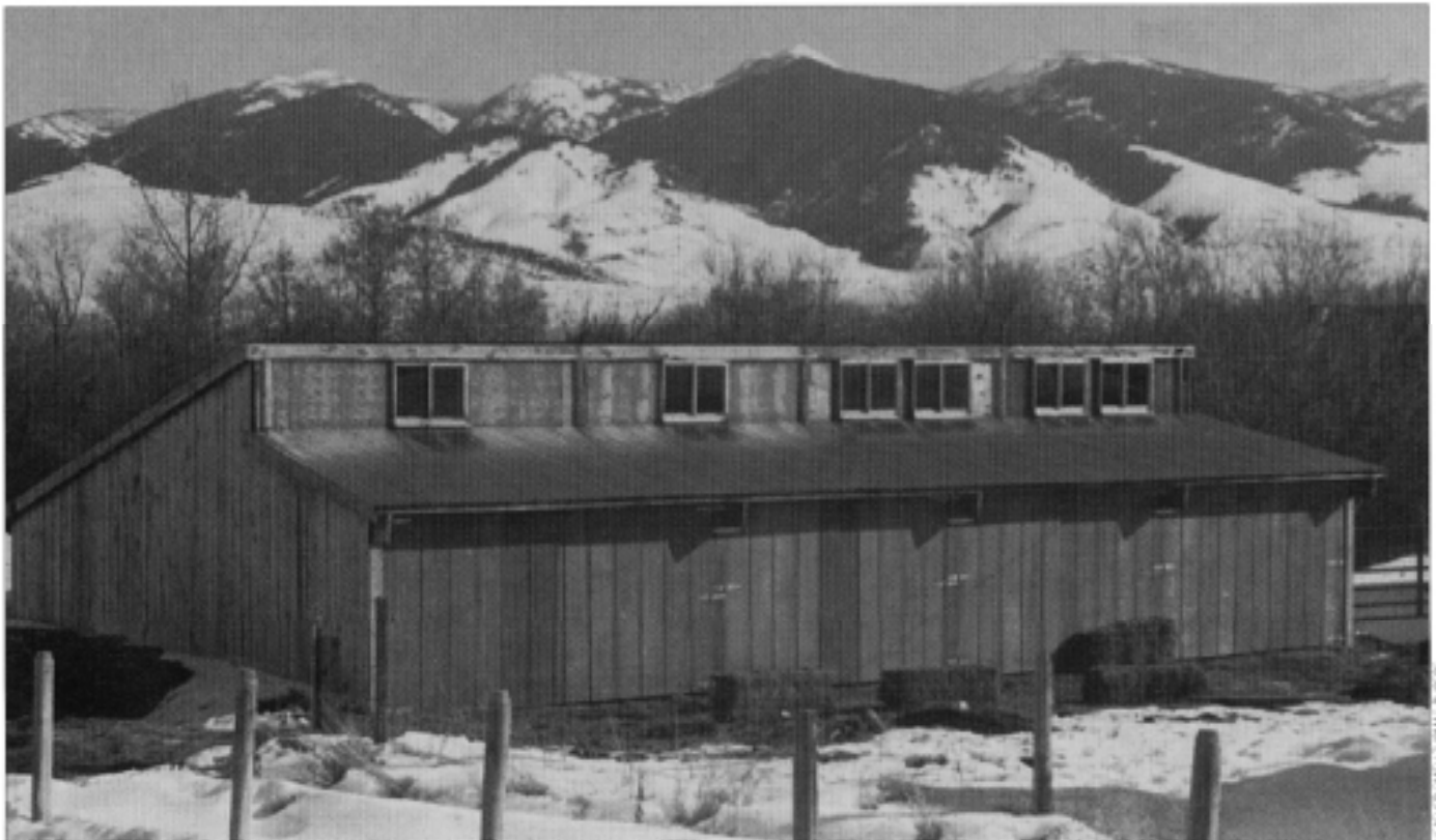
This calving barn was designed and built to stand up against Idaho's toughest winters. It has four rows of stalls and a sloping roof with strategically located windows to gather extra solar heat and light.
