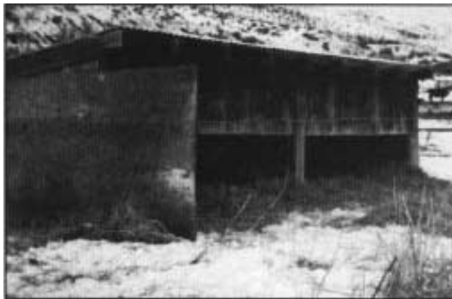
Calf shelters should have a sloping roof, slatted floor with straw bedding, and an opening away from wind.
