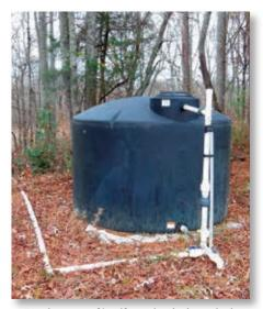
"It takes care of itself. On cloudy days, the battery backup works. We can run the solar-powered system all year round," says Chris Thomas, Hoboken, Ga., who has a 48-volt system that can pump 2-3 gal. per minute into a 200-gal. pressurized tank.
