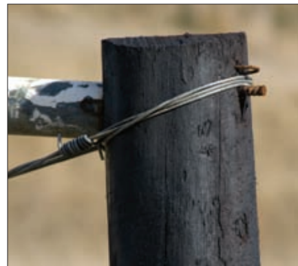
►This closeup shows how a length of rebar or reinforcement rod was used as a pin to hold the horizontal brace pipe at the desired height. About 4 in. of the rod protrudes from the backside of the post and inside the pipe. An inch or so of rod protrudes from the post's nearside, and serves to hold the diagonal brace wire.
