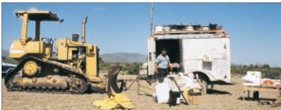
Carlos and Juan spent each day building dirt tanks, or ponds, across this arid ranch. The white trailer was towed behind the dozer between digging jobs. It came complete with cots and "girly calendars" for these heavy-equipment operators. All cooking was obviously done over an open fire.
